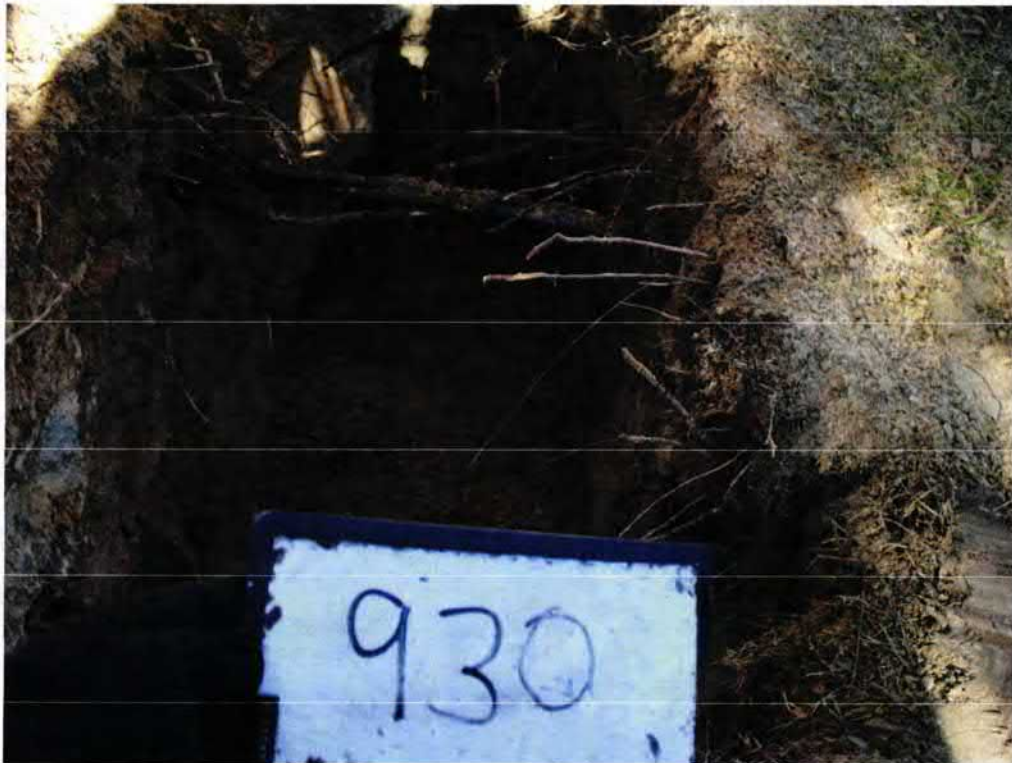
Picture 2: UST 930Albacore excavation.
